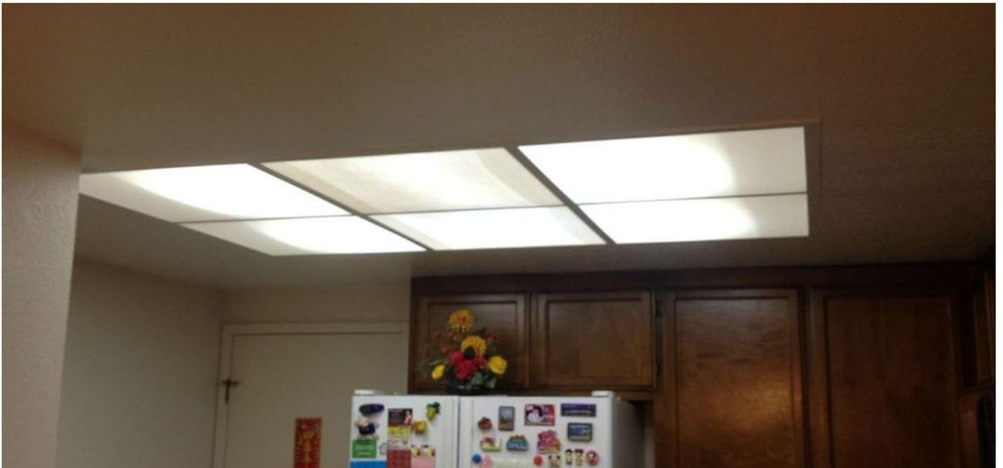
Typically, we can replace ceiling fluorescent light with LED light of half the wattage. To do that, you can choice LED tubes or LED modules.
