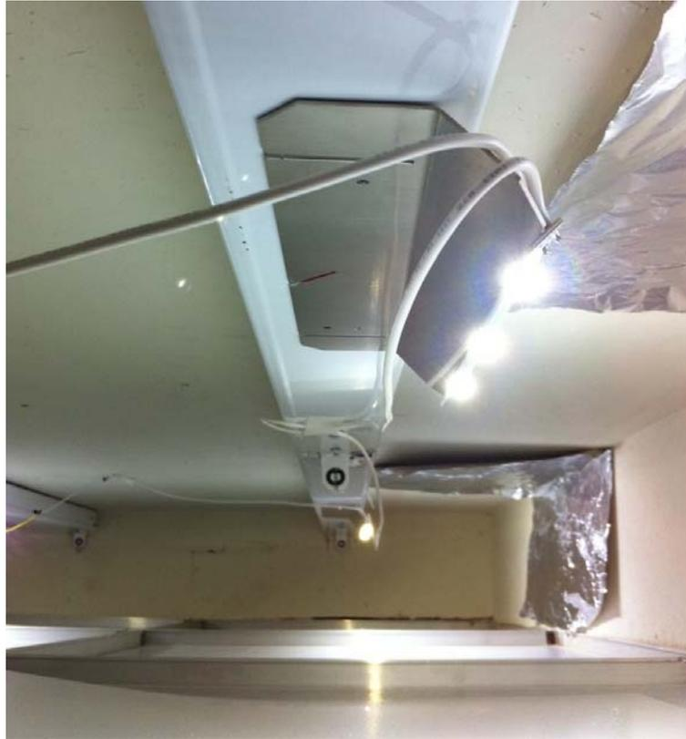
Easy LED module, on the other hand, is mounted in the open, module or LED is working at much lower temperature. Its heat dissipation is so good that a standard 15watt module can take 30 watts of load and work sustainably. Of course we don't recommend such a usage; just let you know that it can take such.
